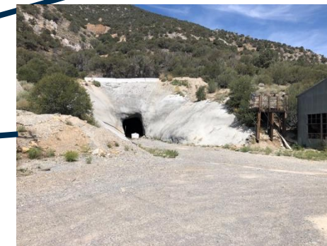
Diamond Tunnel – Portal & Internal
