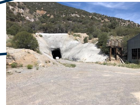
Diamond Tunnel – Portal & Internal
