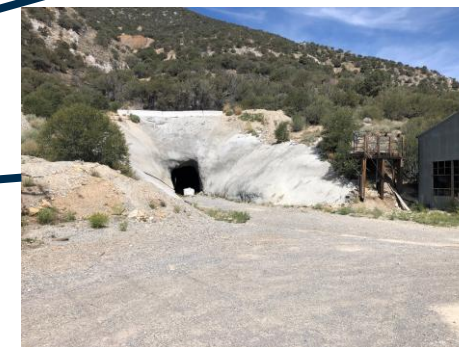
Diamond Tunnel – Portal & Internal
