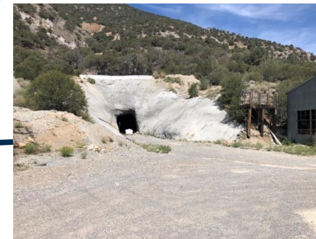
Diamond Tunnel – portal & internal
