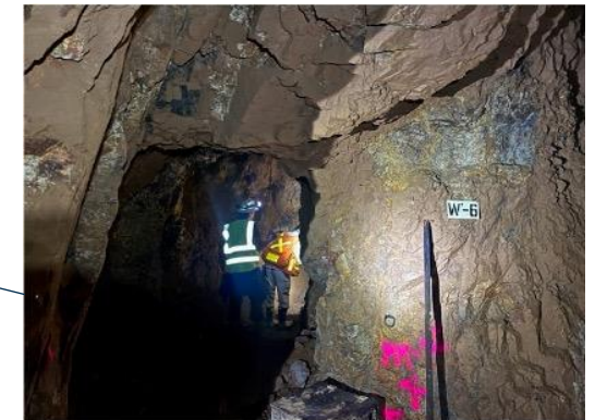
Banner Fault Visible Underground
