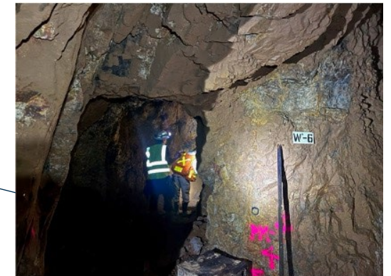
Banner Fault Visible Underground
